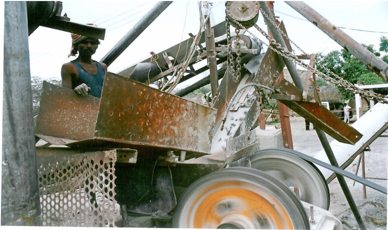
A Close View of Stone Crusher
